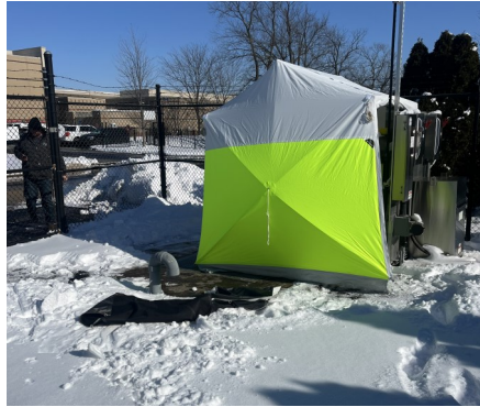
New Tent utilized for cold weather work at Lift Station 20
