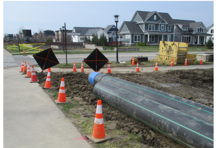
Parallel Lift Station 16 Force Main ready for installation
