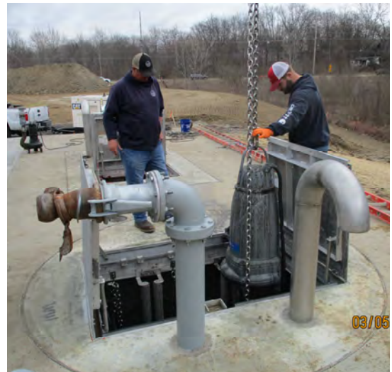
Lift Station 16 New Pump Installation
