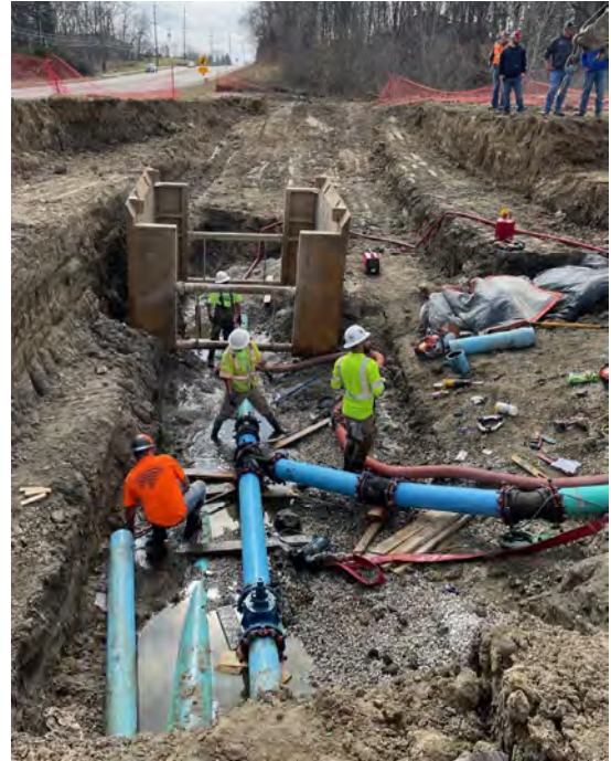
Lift Station 16 Force Main Tie-In
