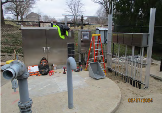
Lift Station 14 Electrical Installation
