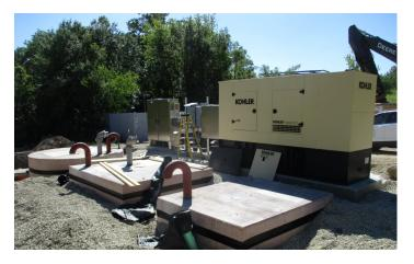
Above: Lift Station #8's new wet well, valve pit, control cabinet and generator.
