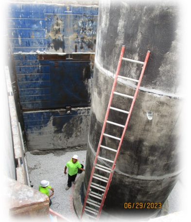
Sealing the structure to prevent I&I
