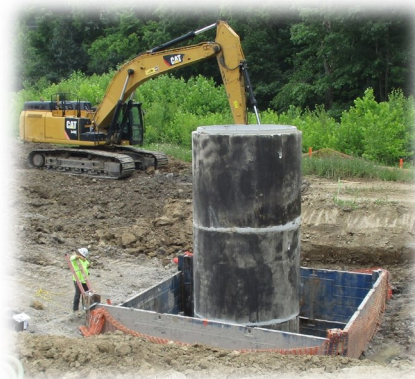
Ottenweller installs the 35 feet deep wet well
