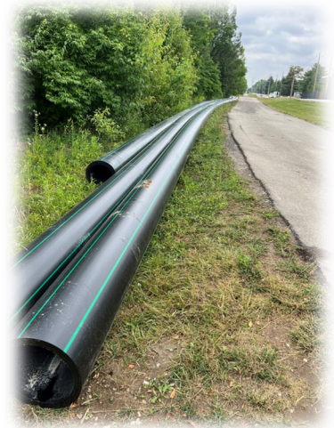
New Force Main Ready to Install Along Ditch Rd.
