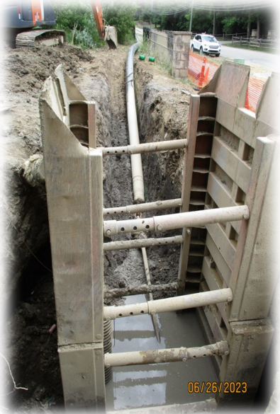
Starting to Pull in New Force Main
